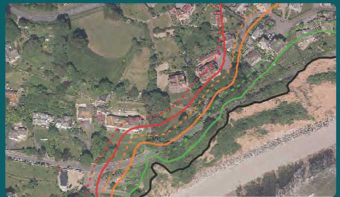
Current cliff position (black line) with predicted cliff retreat and buffer zones over 20, 50 and 100 years
