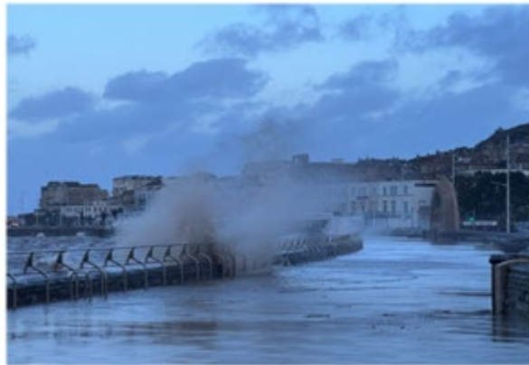
Wave overtopping at Western-super-Mare
